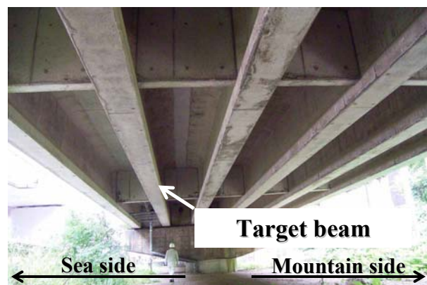
Figure 1: Appearance of PC bridge
