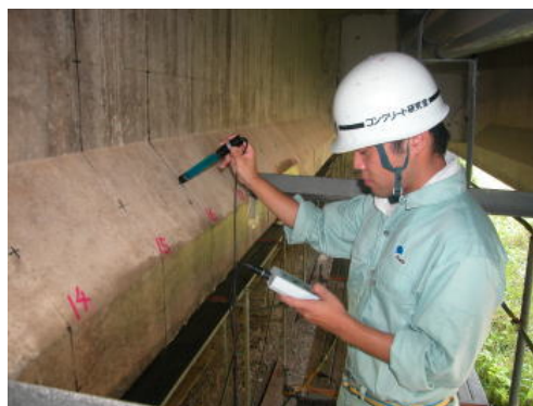
Figure 3: Situation of half-cell potential measurements
